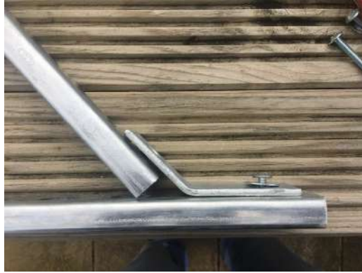
Figure 8: Loosely secure 135° bracket.
