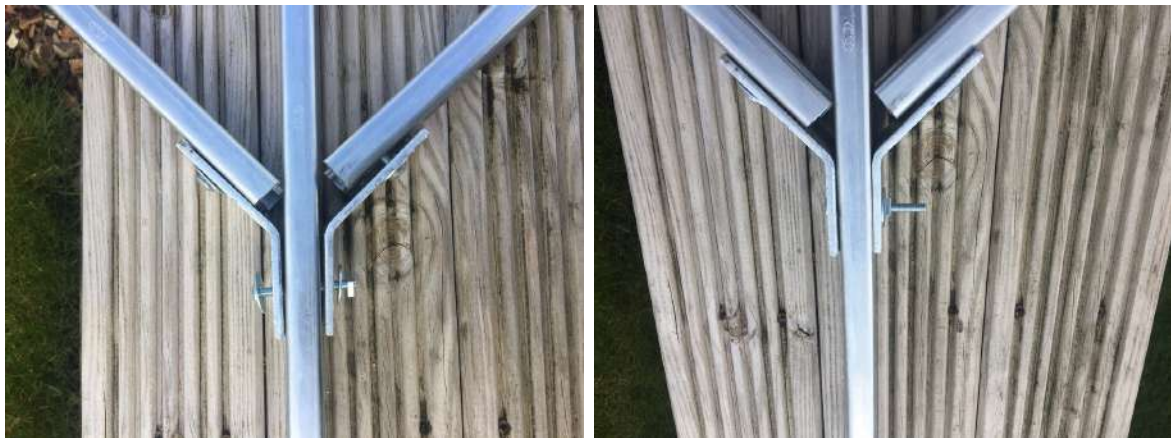
(a) (b) Figure 11: Secure support braces to vertical Unistrut.
