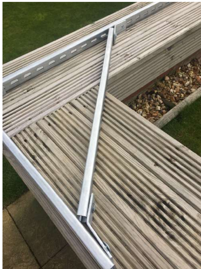
Figure 9: Secure 45° support brace.
